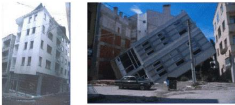
Fig. 5.1.7d Failure of Building Structure Due to Soil Liquefaction, Liquefaction in Izmit, Turkey
